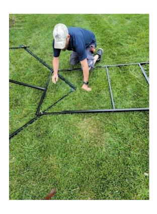
STEP 11: Put the feet on to the Vertical pieces (" the legs"). NOTE: You want to do this now because it is easier to slide on the feet now as opposed to when you stand up the Manger Structure and the Star
