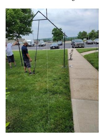
STEP 15: Stake down all the feet (Left, Right and Back). Install the stakes at an angle to help support the feet.
